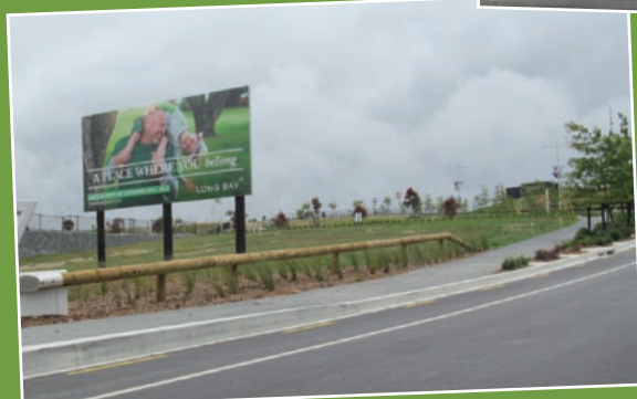
Long Bay Bridge, Auckland
